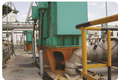
JHB pumps are operating in flue-process at a sulfuric acid plant in Zambia. Capacity: 1600 m 3 /h Head: 25 m
