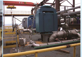
JHB1400-24大型浓硫酸液下泵运用在菲律宾NERIN 2013台金硫酸装置 JHB1400-24 large concentrated acid submerged pumps
