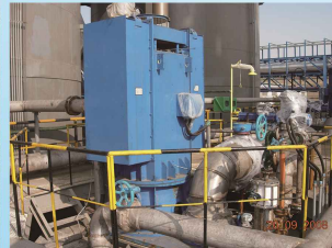
JHB1050-28大型浓硫酸液下泵运用在中色赞比亚谦比希铜冶炼厂硫酸装置 JHB1050-28 large concentrated acid submerged pumps are used
