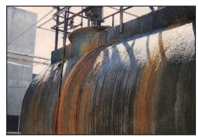
Corroded tanks, containing 98% H<sub>2</sub>SO<sub>4</sub>
