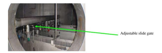
The photo below shows sticks dipped at the end of each the seven troughs in the Drying Tower. The height of the acid in the troughs had a maximum variation around 1/2 inch which equates to a uniform flow with flow variations of less than 5% anywhere in the tower.
