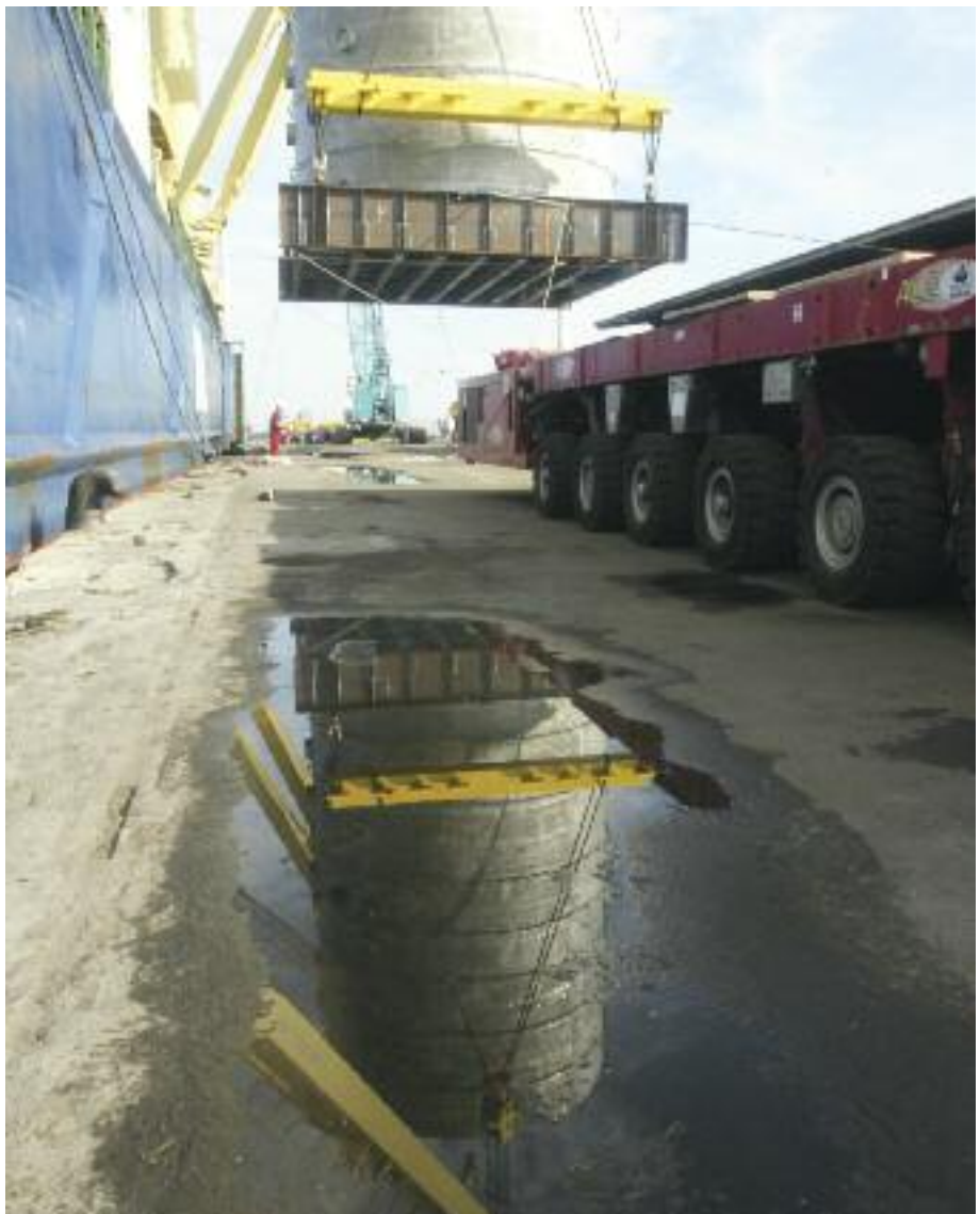
The converter being lifted from the MV Fairlane onto the SPMT at the port of Tamatave.
