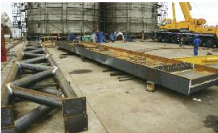
The Bateman Engineering designed stiffening beams and a plate girder that formed part of the lifting beams.
