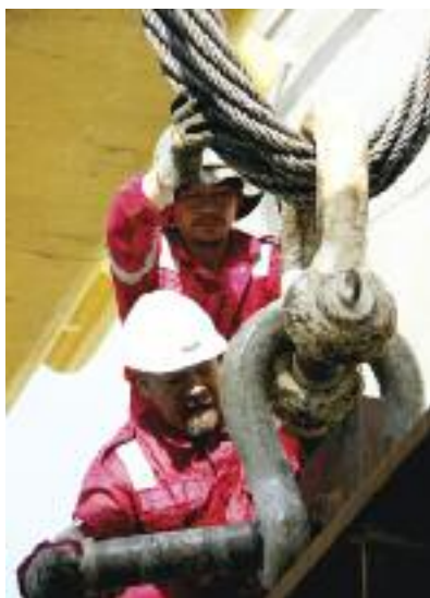
Below: Man-sized shackles for lifting the 395 t converter.
