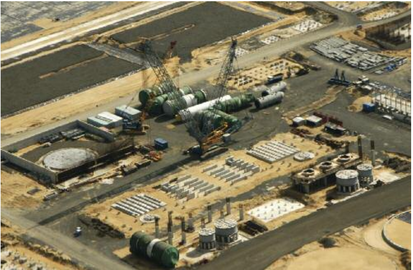
Above: The site ready for the converters.
