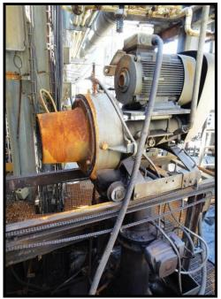
Sulfur Burner (retracted from combustor)
