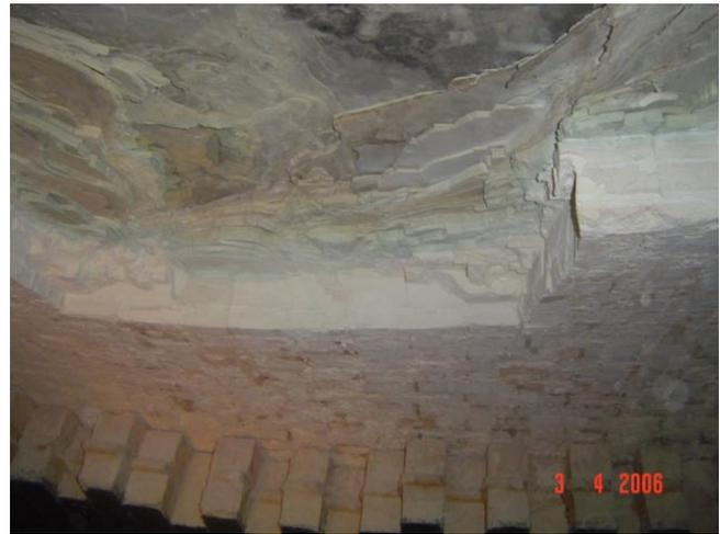
**Fig 3 Sulphur Furnace – Accumulated Sludge**
