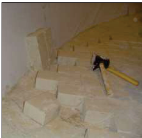
Interface between bottom of the tank and the wall - 90, 65, & 54SG
