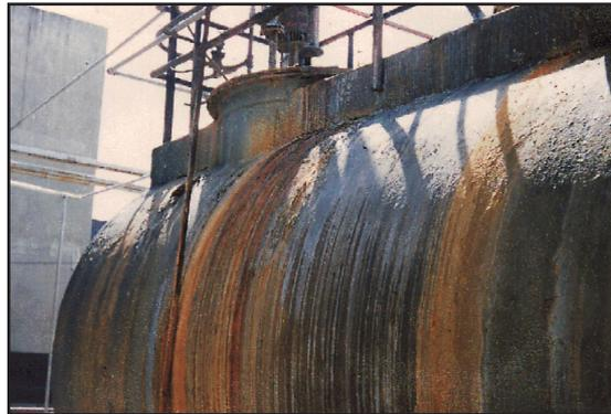
Corroded tanks, containing 98% H<sub>2</sub>SO<sub>4</sub>
