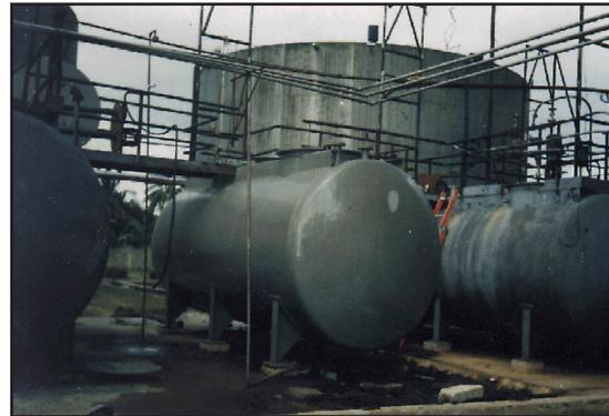
New tanks coated with ARC S4+ internally and ARC S2 externally
