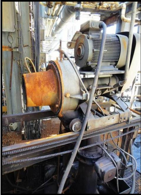
Sulfur Burner (retracted from combustor)
