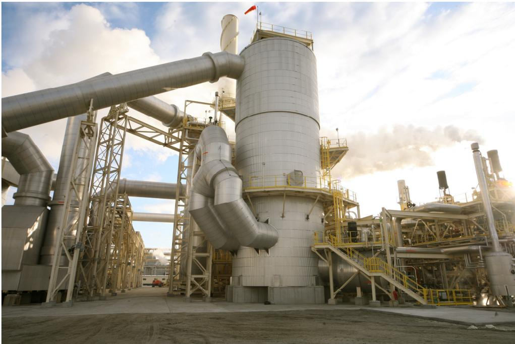
HRS Tower with Steam Injection Duct
