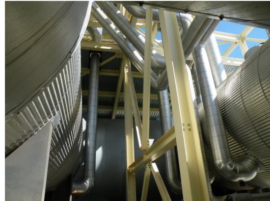
Dual HP Boiler Shells –above is the common steam drum
