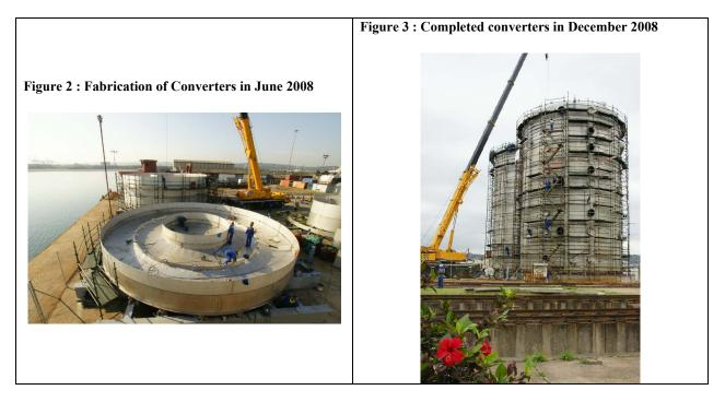
The two converters took Metso ND a total of 65 000 man-hours to complete - all of which were successfully completed injury free. By December 2008 both converters - each weighing 395t, with individual shipping envelopes of 17.8 m by 15.5 m by 24.6 m in heightwas ready for shipment.
